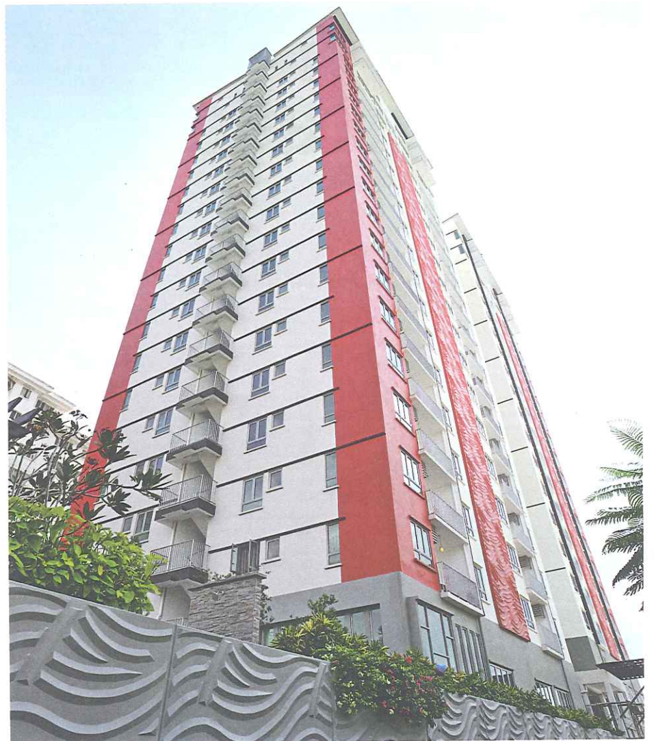
The RM66 mil Puri Tower in Puchong, Selangor
