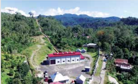
Hydropower Plant at PLTM Bantaeng 1, Sulawesi Selatan, Pulau Sulawesi, Indonesia
