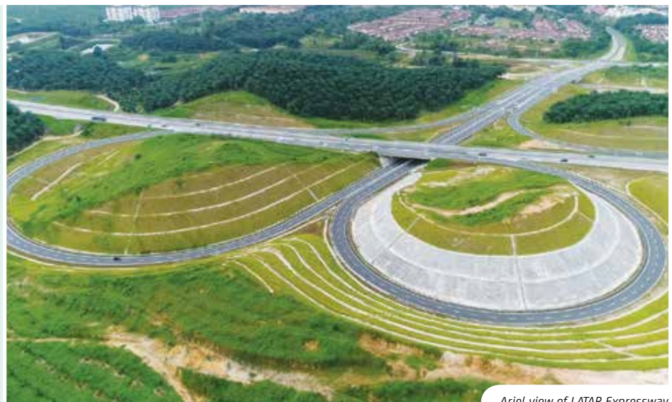
Aerial view of LATAR Expressway
