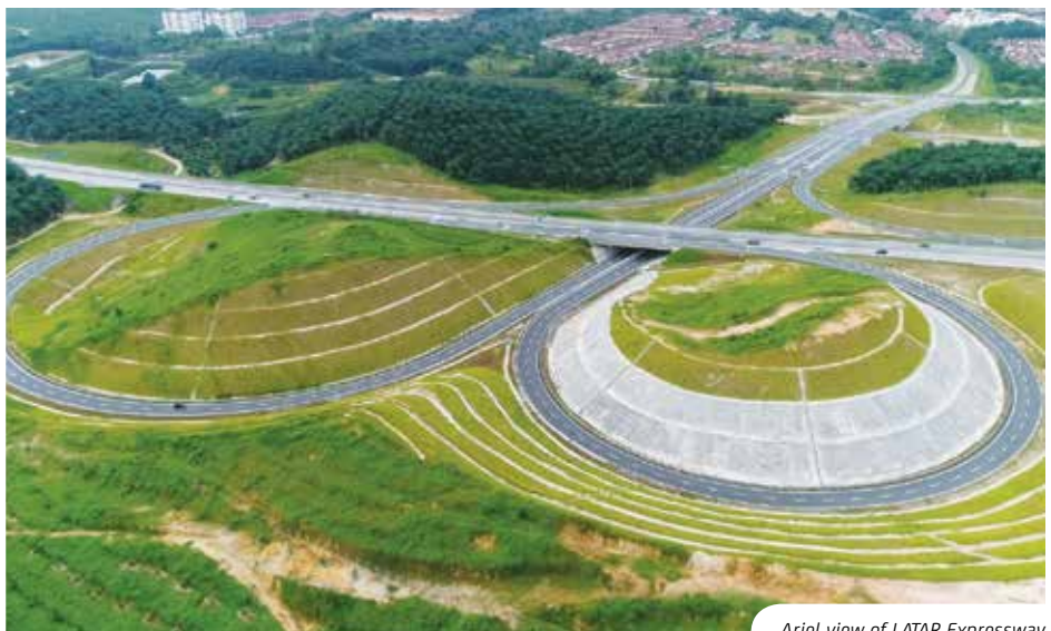
Aerial view of LATAR Expressway
