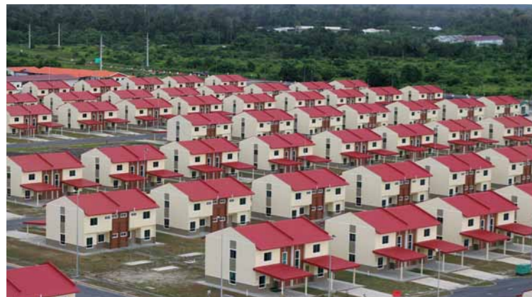
National Housing Scheme in Brunei Darussalam
