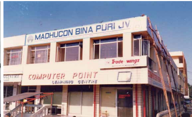
Madhucon Bina Puri office in India
