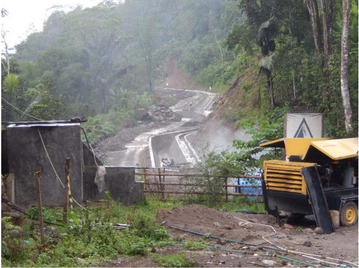
Hydro Power Plant Progress Photos (As at January 2015)
