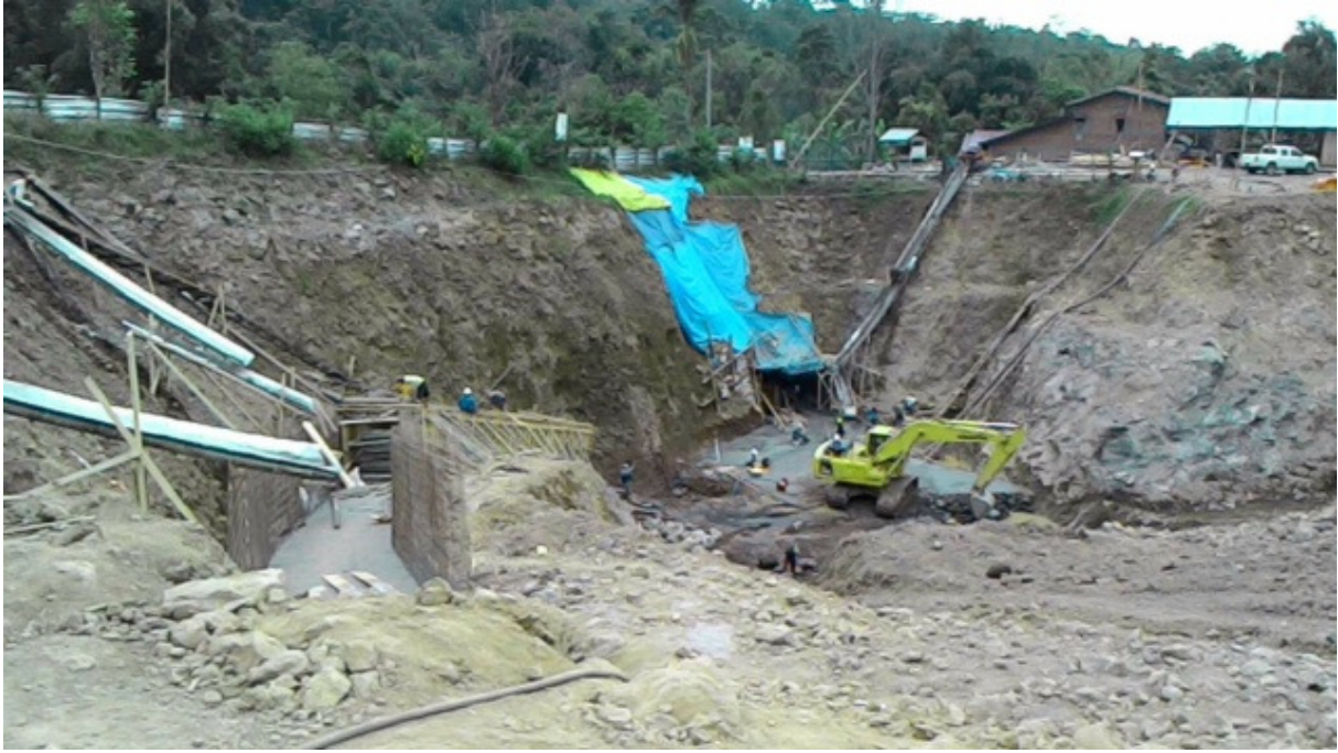
Hydro Power Plant Progress Photos (As at 4 th September 2014)
