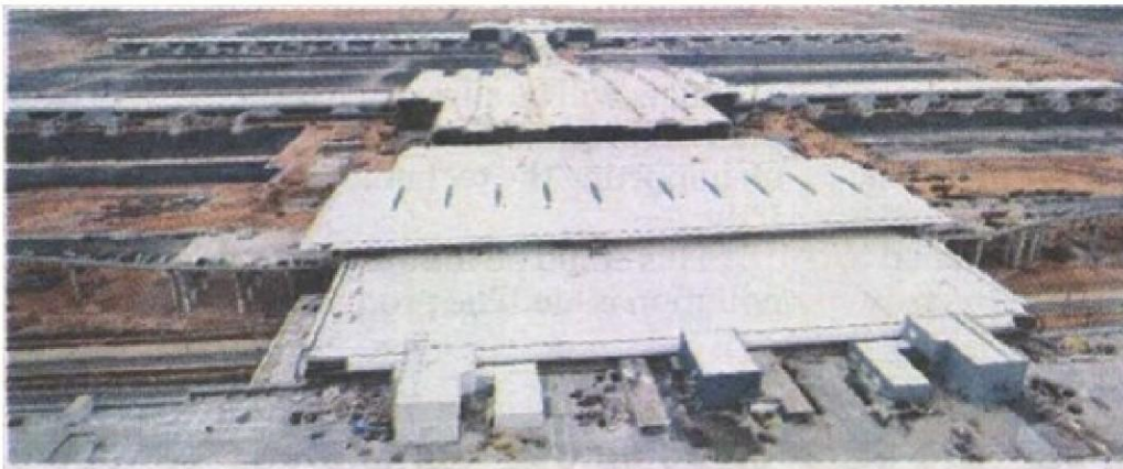
An aerial view of the uncompleted KLIA 2 taken earlier this year.
