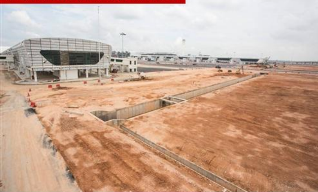
Taxiway and Parking Apron at S1 & S5 (By Other Contractors)
