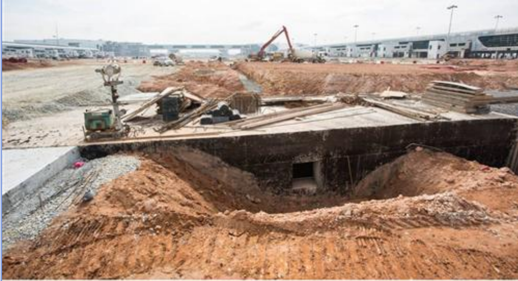
Taxiway Connect To New Runway (By Other Contractors)
