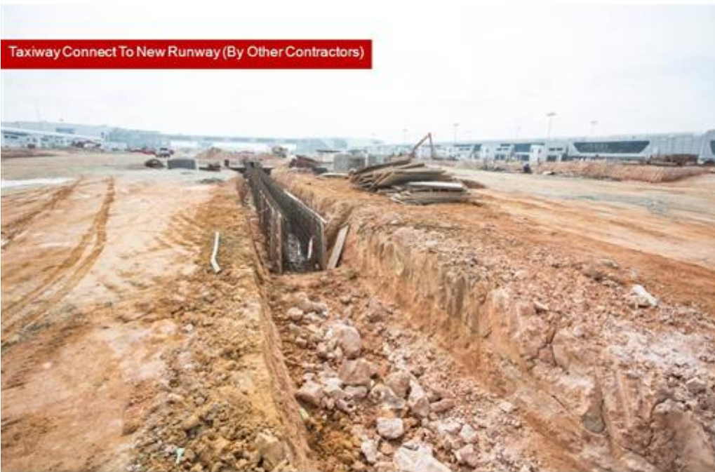
Taxiway Connect To New Runway (By Other Contractors)
