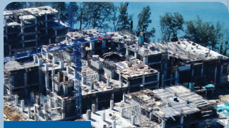
Construction in progress
