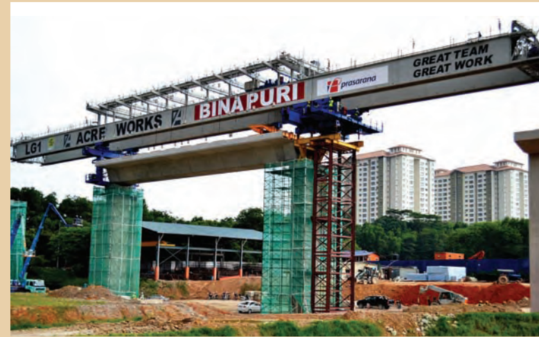
Ampang Light Rail Transportation Package A (LRTA : AMG)
