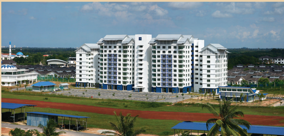
Kem Batalion 6 (PGA) Polis DiRaja Malaysia (PDRM), Muar, Johor ■ Completed in December 2011 ■ Contract value: RM300 million (USD96.7 million)
