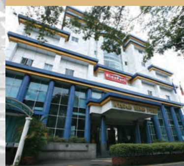
Wisma Bina Puri, Corporate Office in Selayang
