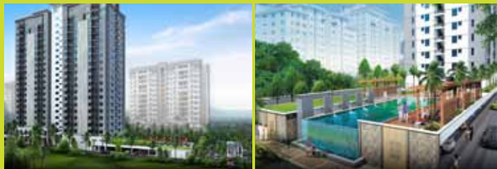
The Puri Tower, Bandar Bukit Puchong
