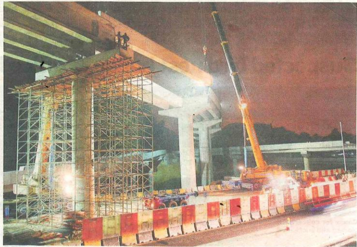
Smoother travel: The dual-carriageway links Templer's Park in Gombak district to Ijok in Kuala Selangor.
