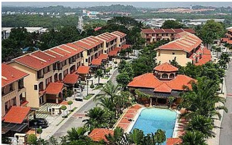
An aerial view of Bina Puri Holdings Bhd's Taman Villamas project in Sungai Buloh, Selangor.
