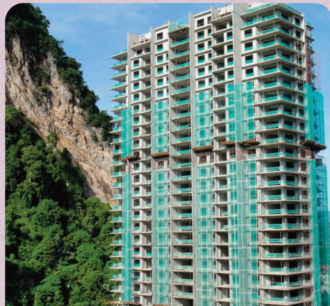
Current on going construction activities
