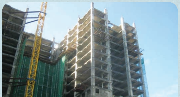
Current on going construction activities
