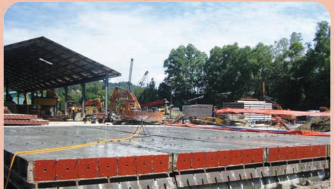
Current on going construction activities
