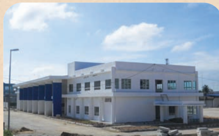
Current on going construction activities
