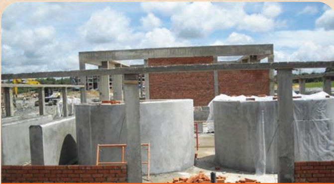
Current on going construction activities
