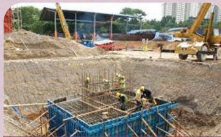
Current on going construction activities
