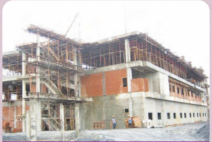
Current on going construction activities
