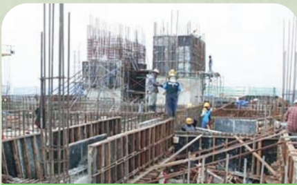
Current on going construction activities
