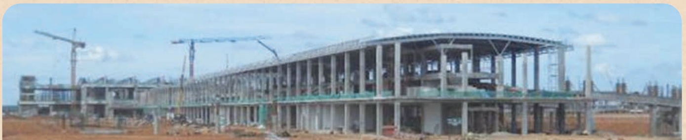
Current on going construction activities
