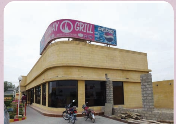
Soon to be upgraded, temporary 'rest and service' area at the Karachi-Hyderabad Highway
