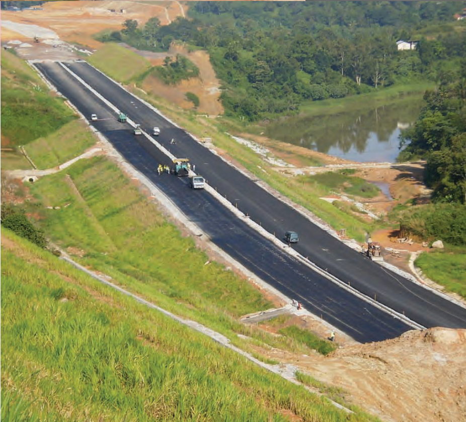
Laying works is on progress
